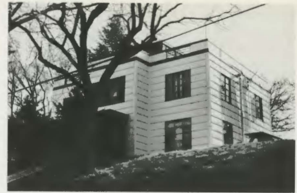
Armco-Ferro-Mayflower House (01003) The house was produced by two Ohio steel companies, the American Rolling Mill Company and the Ferro Enamel Corporation to illustrate their new frameless steel construction.
