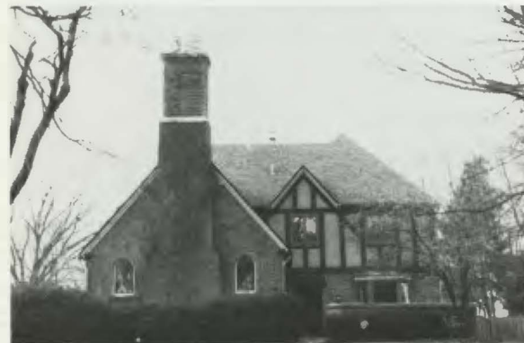
Tudor Revival: House, Valparaiso. 32050
