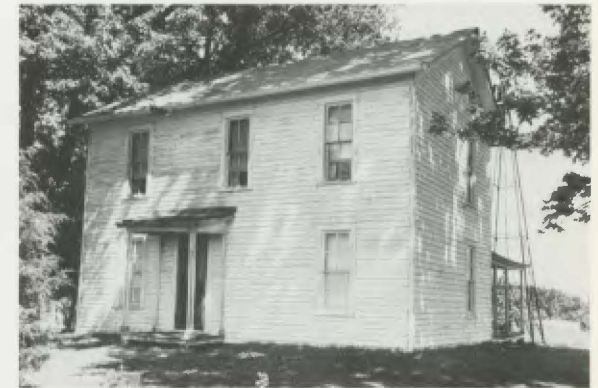
I-house: Henderlong House, Union Township. 35020
