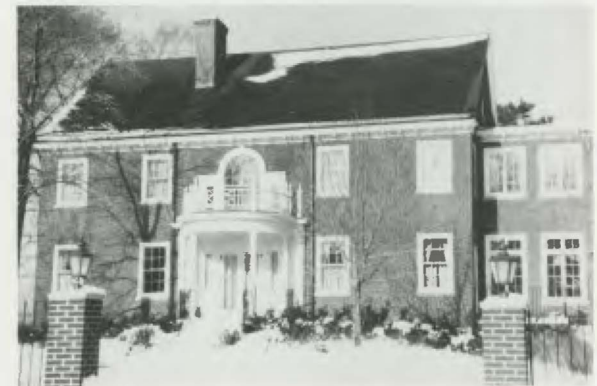
Colonial Revival: House, Ogden Dunes. 11001
