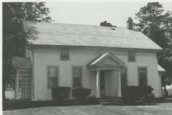
Central-passage: House, Porter Township. 40005
