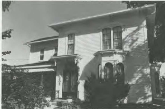
Lorenzo Freeman House (32066) A section of the house was built in 1849 for Lorenzo Freeman, a local businessman.
