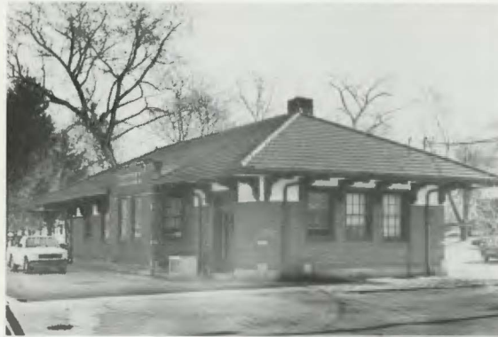
Chesterton New York Central Passenger Depot (09011) The depot was built in 1914 for use as a passenger station. It is now used as offices for a local utility company.
