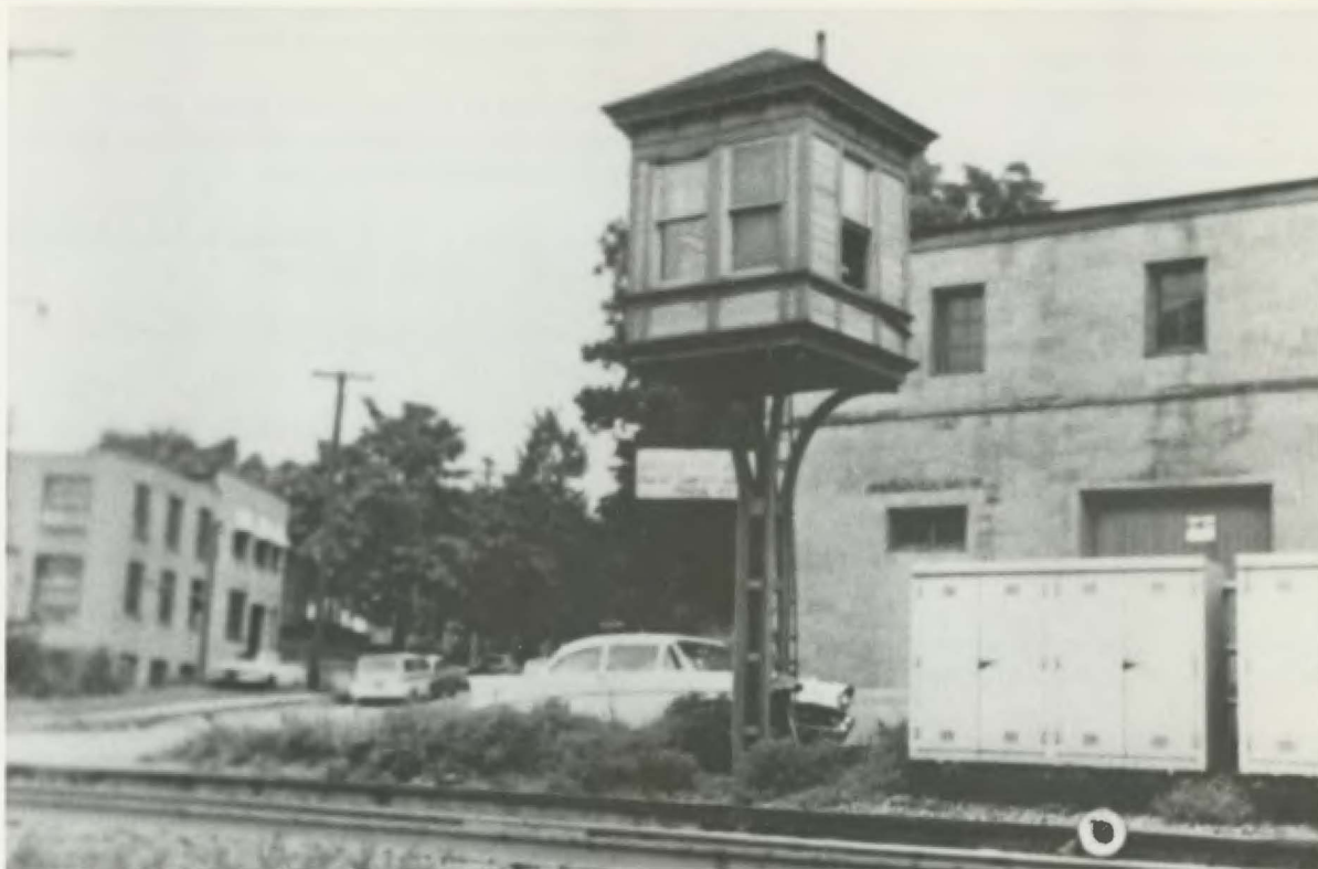
Switch Tower, Valparaiso. Courtesy: George E. Neeley.
