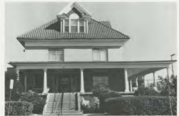
Dr. David J. Loring House (32063) In 1906 Dr. David J. Loring commissioned local architect Charles Lembke to design a building to serve as a house and medical clinic. Loring was a physician and surgeon and served as vice present of the Indiana State Medical Association and was the founder of the Porter County Medical Society. The house is currently owned by the Valparaiso Women's Club. It was listed in the National Register of Historic Places in 1985.
