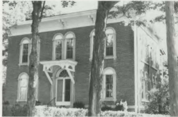
Double-pile: House, Valparaiso. 34046
