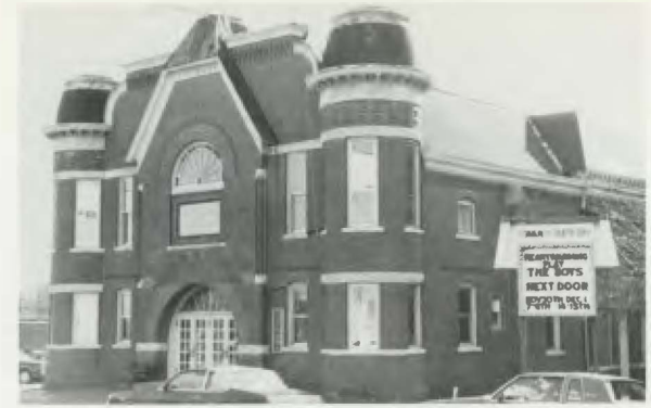
Memorial Hall (31071) The hall was designed in 1893 by noted local architect Charles Frederick Lembke in memory of Civil War veterans. The 1000 seat hall was to be used for patriotic rallies, concerts and lectures. The building played host to such luminaries as William Jennings Bryan, Theodore Roosevelt, John Phillip Sousa and the Marx Brothers. The hall is now used by a community theater group. It was individually listed in the National Register of Historic Places in 1984.
