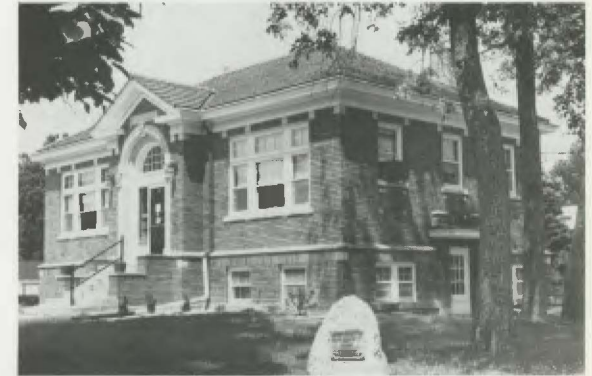
Neoclassical: Hebron Carnegie Library, Hebron. 56023
