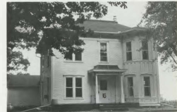
John Wallace Rigg House (40011) This house, also known as "Forest Home" was built in 1884. Rigg, a farmer, raised 12 children in this house. He also served as the Porter township trustee for nine years.
