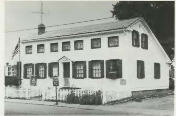
Saltbox: McCune House, Hebron. 56012
